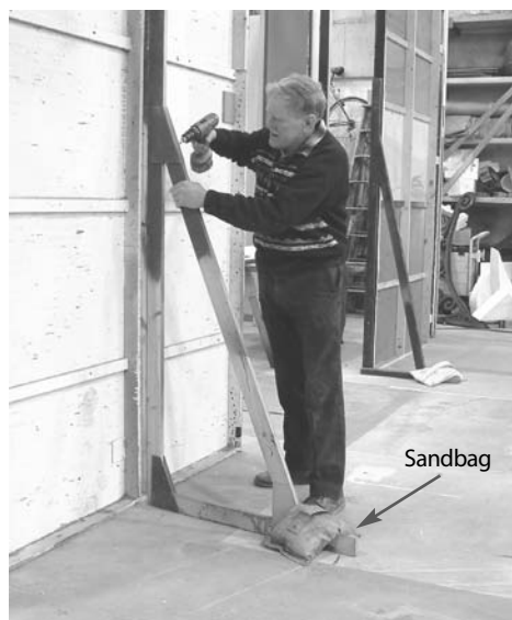
Ken Manning repairs a French brace. Note the placement of the sandbag. Australian Film Television and Radio School.
